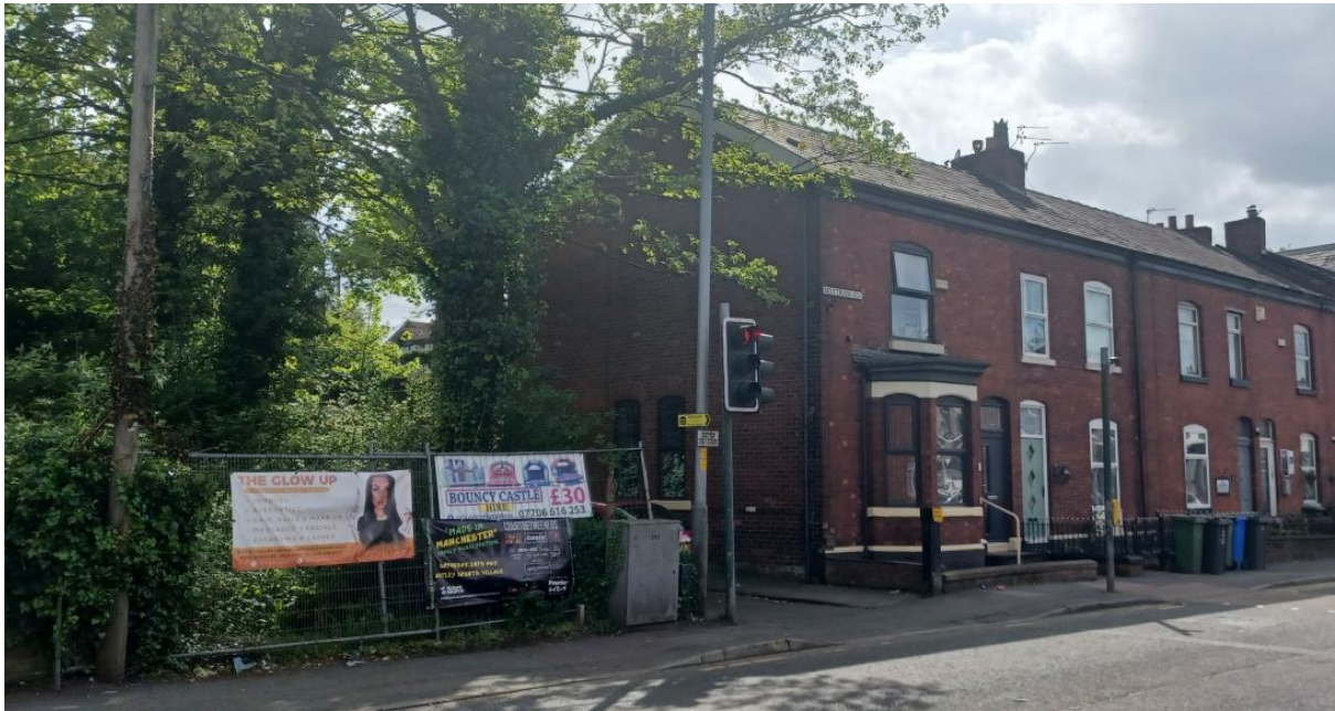
Photo 2: Mottram Road Frontage (1)
