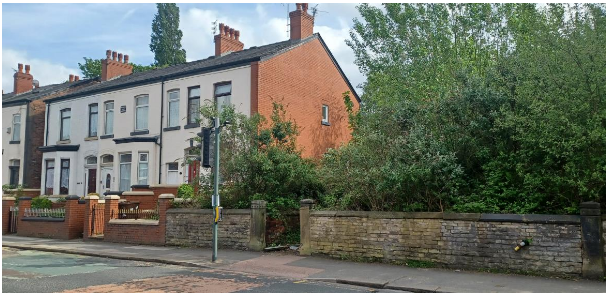
Photo 3: Mottram Road Frontage (2)
